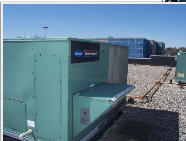
Roof Top HVAC unit replacement and automation
